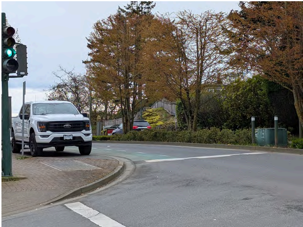
Figure 4.9: Site Visit Photo – Parked Vehicle Obscuring Sight Line at Island Highway & Stormont Road
